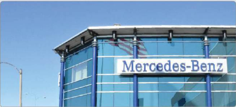
Mercedes Benz of Boston Renovation
